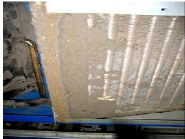
Clogged condenser coil.
